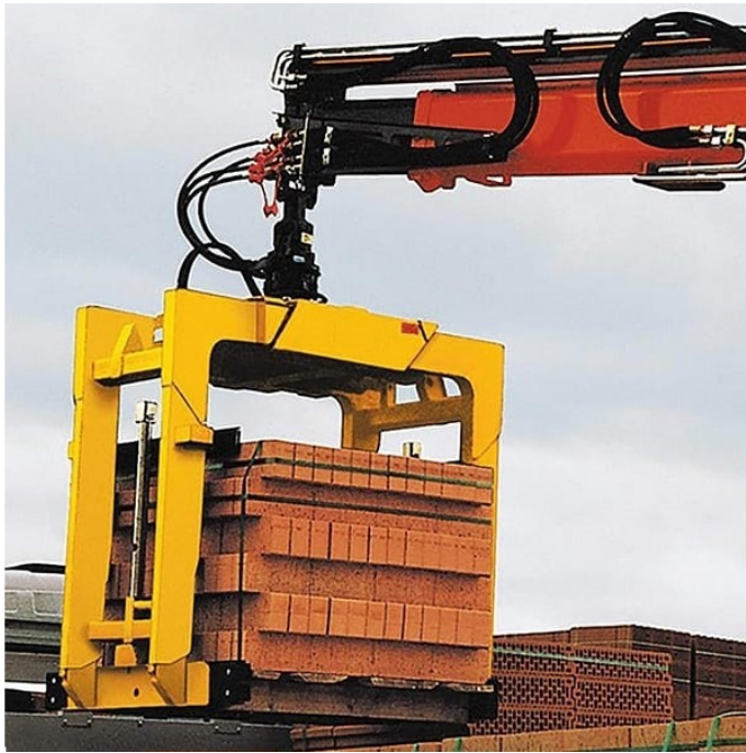
Image 1. Example of grab handling of a palletized unit load at a construction site.
