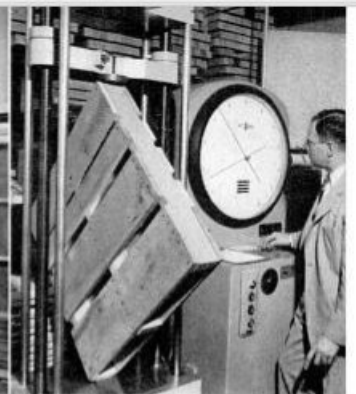
"IF YOU WANT TO MAKE a good pallet, you have to use a good nail," says Stern, here testing a pallet's rigidity on a machine that applies pressures of 10 to 12,000 pounds.
