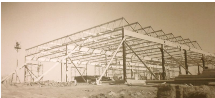
Photo: The Brooks Center under construction.
